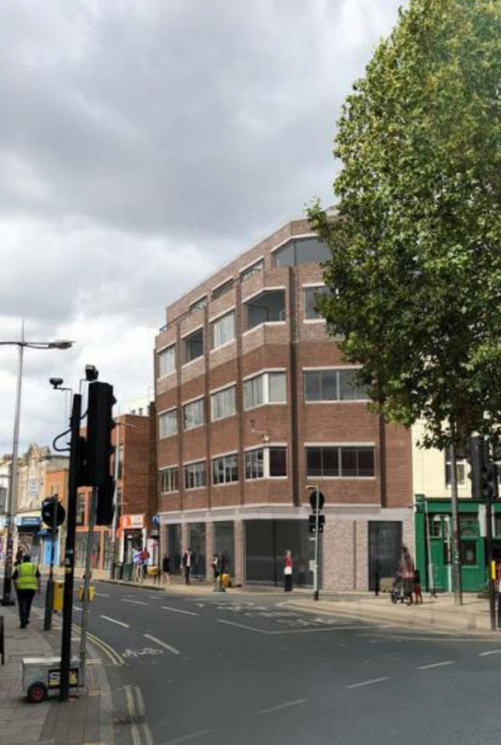
View of the new proposal for 223 Rye Lane showing additional 3 storeys on top
